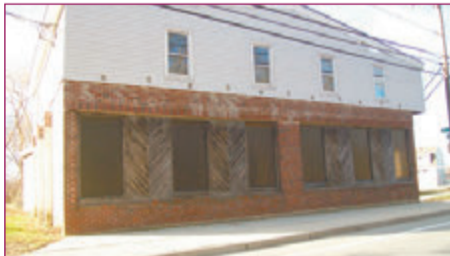
Tiverton - Busy Main Road location; high visibility. Solid commercial building with loading dock. Many possibilities. $169,000
