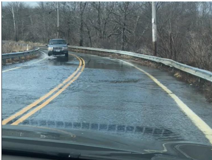
Figure 6: Schoolhouse Rd flooding during rain event (March 2018)
