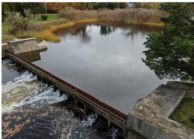
Figure 2: Lower Kickemuit Reservoir Dam: Tidal flooding of lower impoundment (in foreground) during a moon tide
