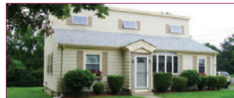
Tiverton - Beautifully maintained Cape with open floor plan, hardwoods, 1st floor bedroom. Large expanded second floor includes in-law set up. Well landscaped yard, large mahogany deck, shed and oversized garage. $299,000
