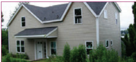
TIVERTON - Nice waterfronts of Mount Hope Bay located across the street from the water. The interior is in unfinished condition (rough framing only). Walk-out lower level. Good opportunity for builder to finish. $269,000
