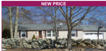
Tiverton - Turn key ranch in bucolic So. Tiverton. 1,128 s.f., 3BR/2Ba, attached garage, finished walkout basement with extra room for den/office. Stonewalls, decking, overlooking 1 acre lot. Natural surroundings, Close to Tiverton 4 Corners and highways. New Price $319,000
