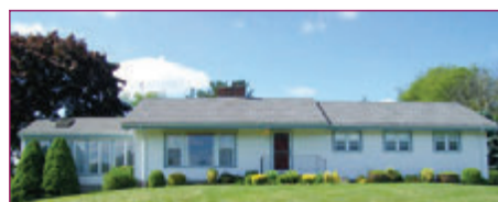
Tiverton - Spacious one level living off Nanaquaket Rd. 3 bed, 2 bath Ranch with large sunroom addition & cathedral ceilings. Hardwoods, fireplace, 2 car integral garage. Well landscaped acre + in private setting. $399,000
