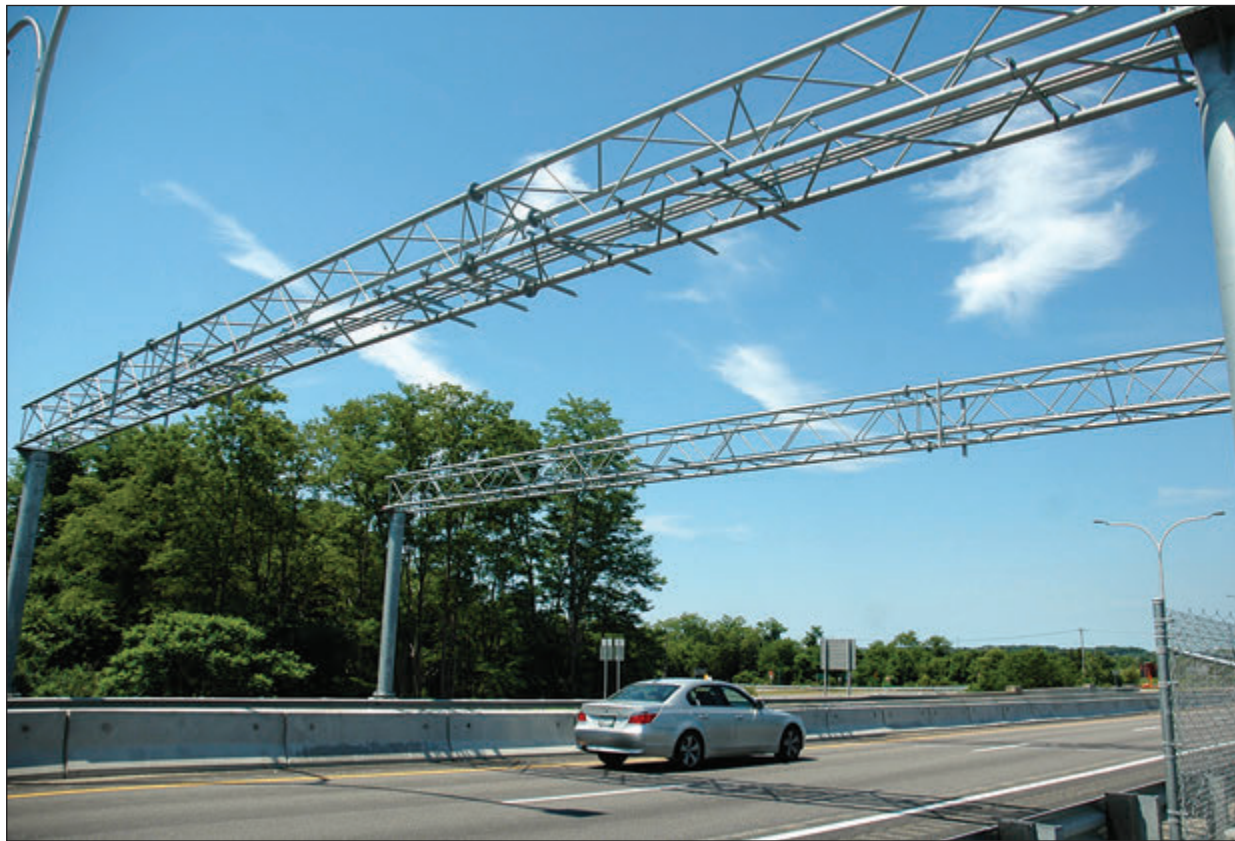
The toll gantry remains but has been stripped of its electronic equipment after tolling ended on the Sakonnet River Bridge last week.
