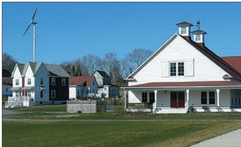
Sandywoods Center for the Arts, several of its residences, and a wind turbine.
