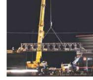
In this Aug. 1 file photo, cars and trucks stream by as workers from WSDOT's emergency contractor, Guy F. Atkinson Construction, guide a 50-foot temporary steel bridge into place over the damaged Chamber Way overpass in Chehalis.
