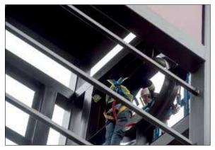
A pair of workers drill holes in the new clock tower as they attach panels onto the structure along the Gordon Aadland Esplanade on the Centralia College campus on Wednesday
